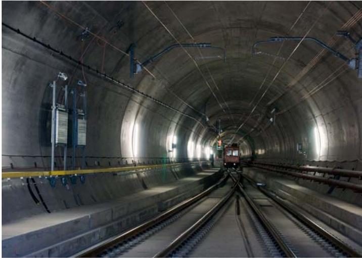
After 20 years in the making, Switzerland's Gotthard Base Tunnel opened last Wednesday to much fanfare. Now the world's longest rail tunnel, the Gotthard has a route length of 35.5 miles and a total of 94.3 miles of tunnels, shafts, and passages. The largest construction project in Swiss history, the €11bn tunnel is also the world's deepest, running more than 1.4 miles below the Swiss Alps. Unfortunately, the project's opening ceremony also reached great depths — of depravity.
